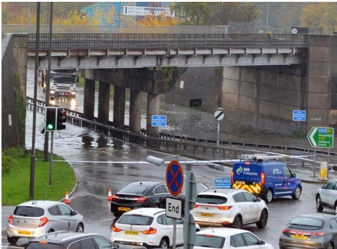
Figure 26: Horns Bridge, Chesterfield Flooded
